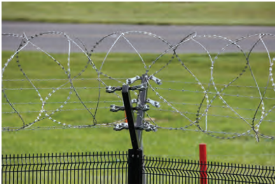
Fig. 4.6: Barbed wire and electric fence
