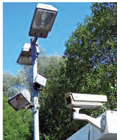
Fig. 3.9: Security lighting system with CCTV camera
